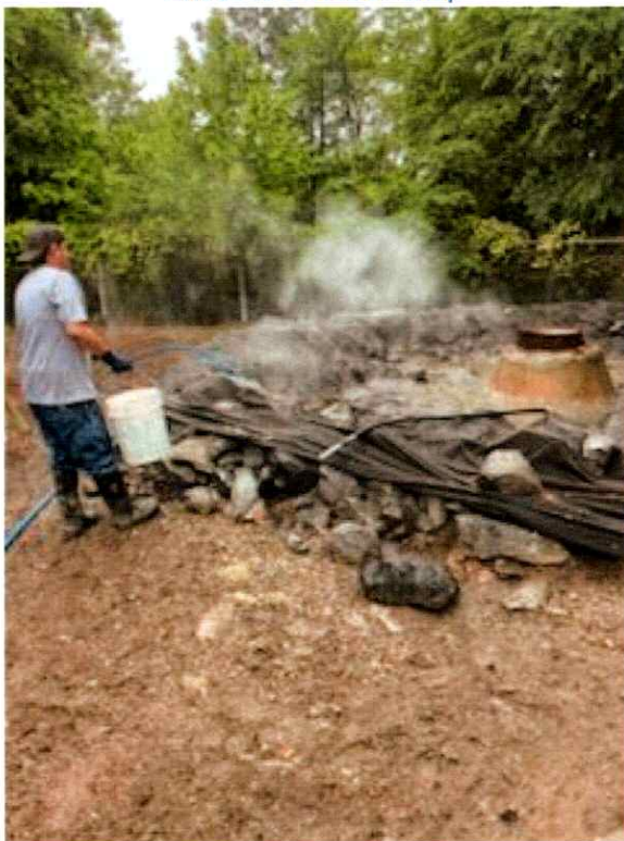
MH 1866 During Cleanup
