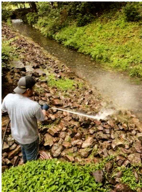
MH 3728 During Cleanup
