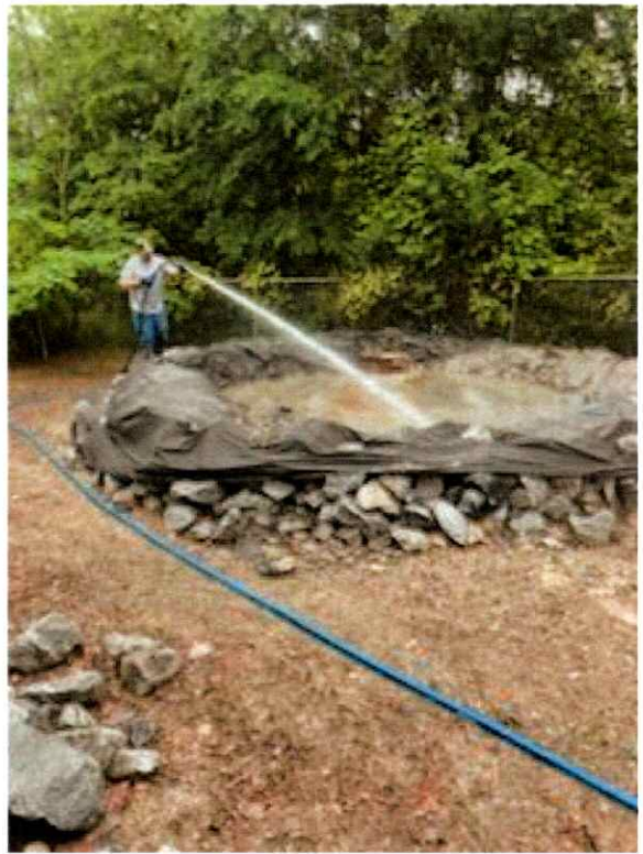
MH 1866 During cleanup
