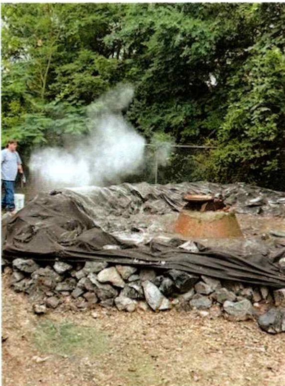
MH 1866 During Cleanup
